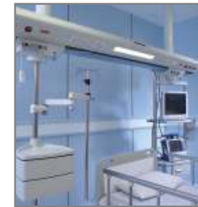
Ceiling Supply Beams
